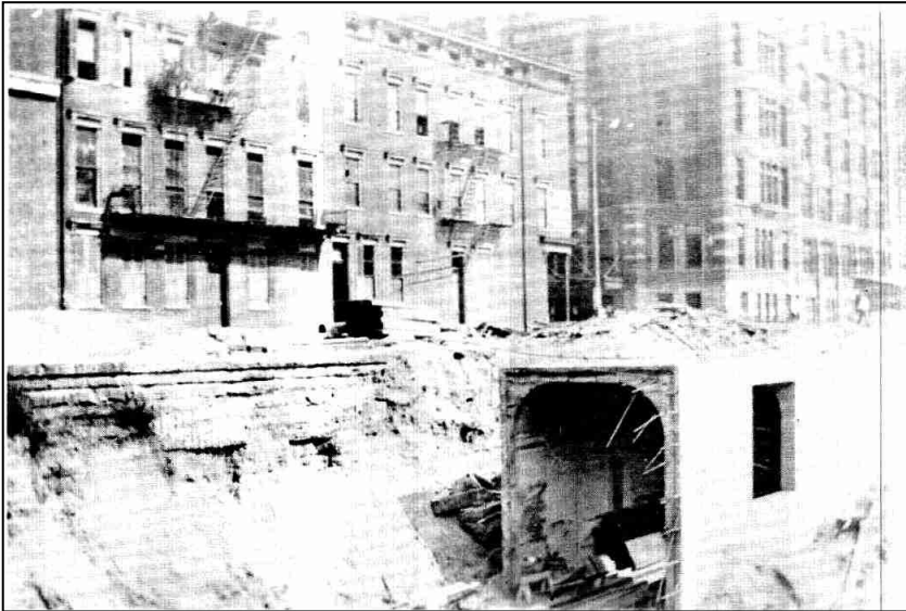
Early Subway Tunnel Construction at Central Parkway
