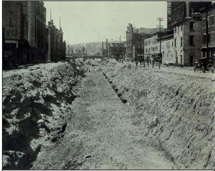
More Early Subway Tunnel Construction
